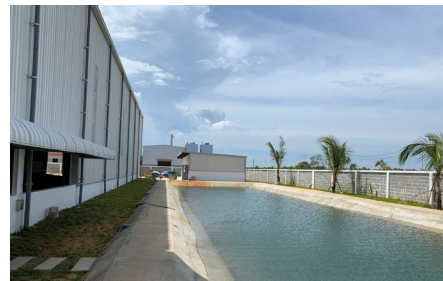
Picture 2: The wastewater system at the new, “green” production facility in Vietnam supplies purified, drinkable water. Source 2: Wendler Interlining Group, publication free of charge
